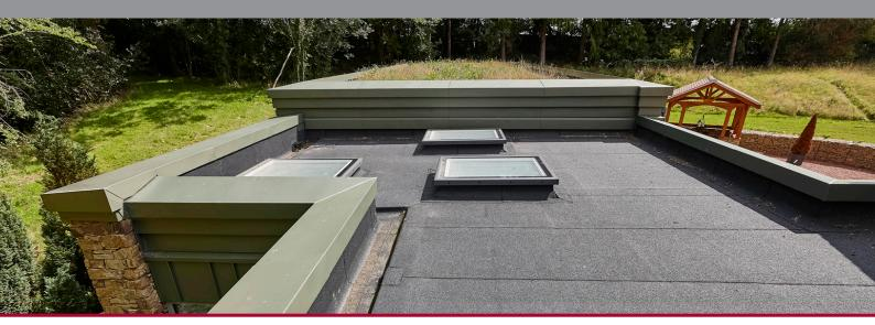
originally specified as a zinc but again due to compatibility issues and to reduce costs this was amended to the SIGnature bituminous membrane used on the larger flat roof area.
