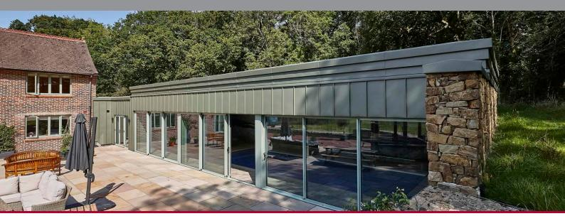
The dark brick plinth and green zinc cladding have been used to blend the extension with the grass. Meanwhile, the walls have been built in natural stone gabions which over time will weather and blend in with the clay ground.
