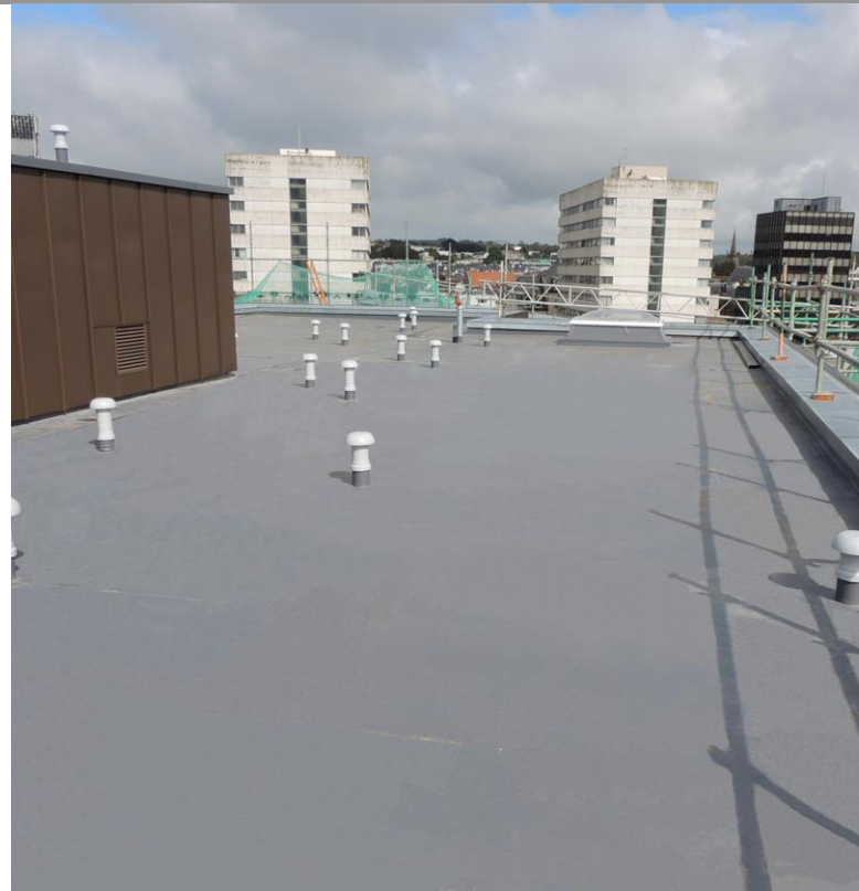
Armourplan PSG system was chosen to waterproof 800 m 2 of the main roof area.
