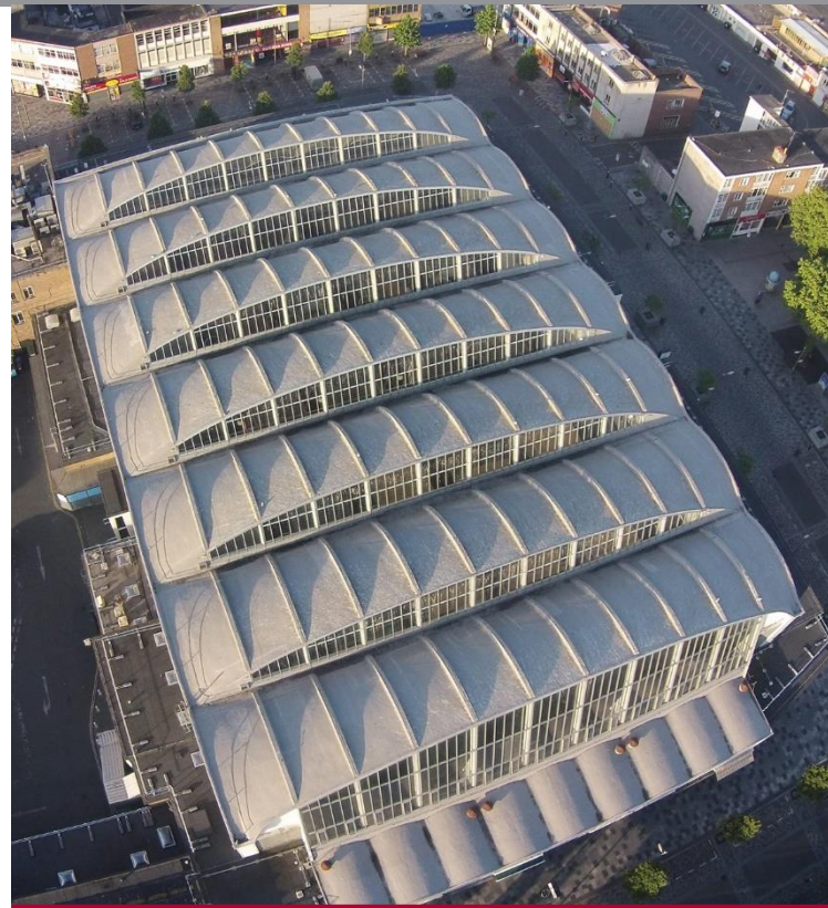
AH-25 provided the perfect solutions, allowing traders to continue "business as usual" while roofing work was in progress
