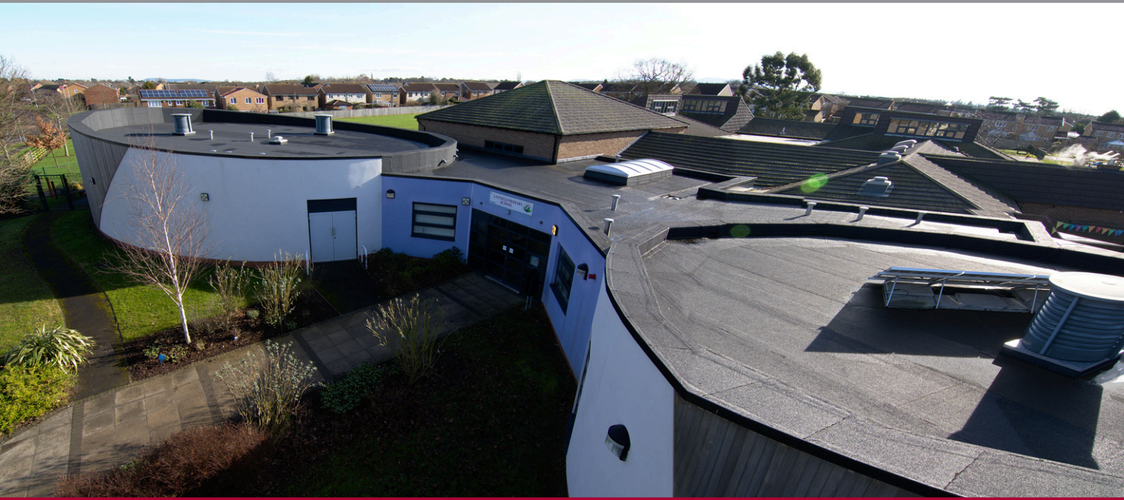
The new overlaid roof at Layfield Primary
