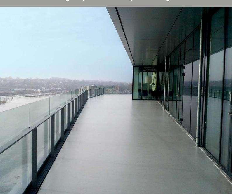
A unique liquid waterproofing system based on a polyurethane-modified methylmethacrylate. This combination assures that the finished system is rapidly ready for use and can also be applied during the winter period at very low temperatures.
