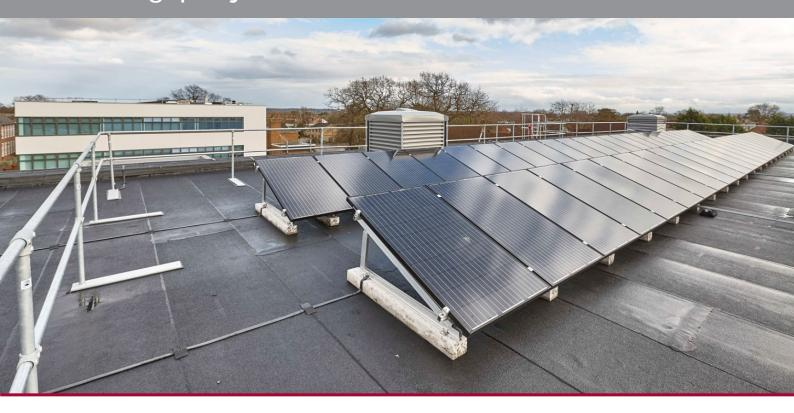
deck, the bitumen primer required for the felt vapour control layer would stain the decking webs and with no ceiling, this would be unsightly. SIG negotiated a hybrid system with our partnering manufacturer comprising a robust, cost effective, reinforced bituminous membranes with a polyethylene VCL to solve acoustic and aesthetic issues.
