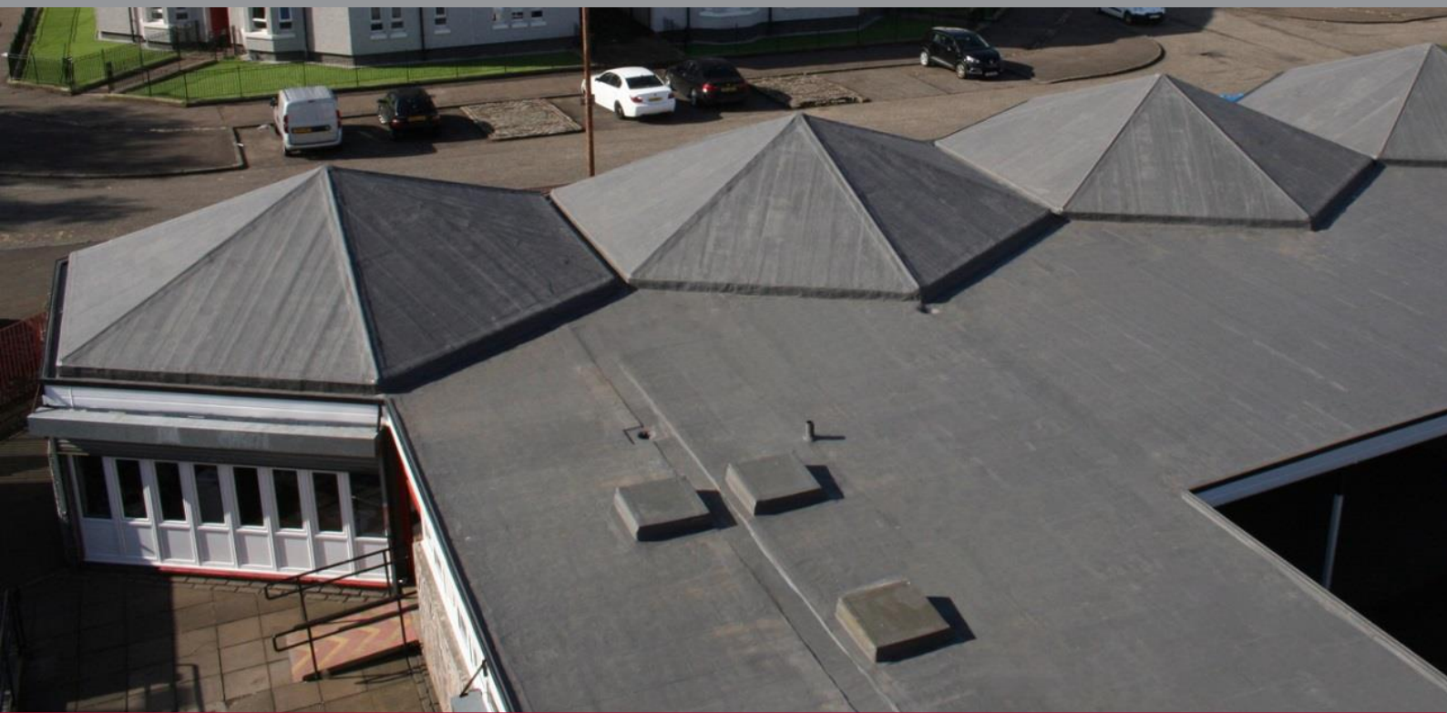
Sacred Heart Primary School, Glasgow 450m 2 of roof refurbished in AH-25
