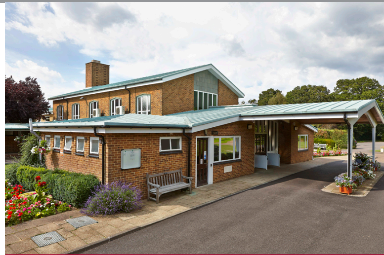
The use of Rhepanol fk roofing membrane finished with copper roof paint maintains the traditional appearance while dealing effectively with the threat of theft.
