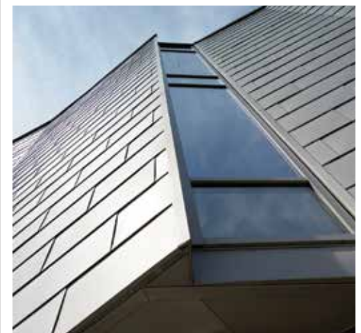
Top The front elevation of Northbrook College's new learning centre framed in its zinc shingle skin.
