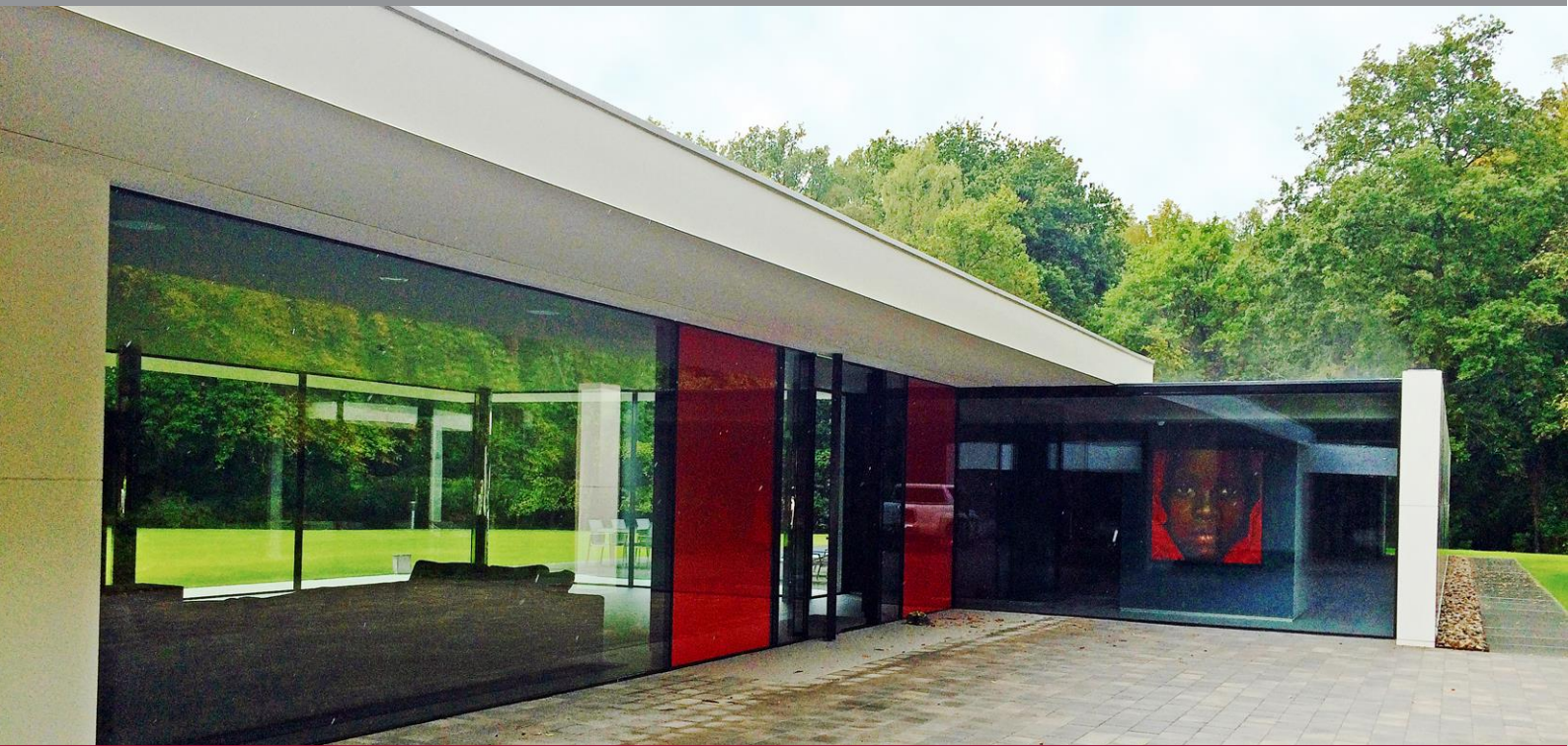
Front elevation of the property showing the minimalist requirement for the flat roof application
