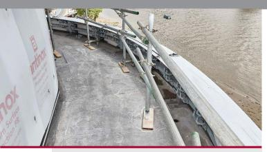
A sheet membrane solution would have been excessively complicated, whereas a liquid becomes homogenous. The Hydrostop AH+ waterproofing would be hidden behind the cladding; so roofing contractors, Knight Asphalte had to be confident in its performance.
