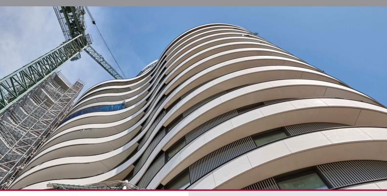
SIG Design Technology's Hydrostop AH+ liquid system was chosen as the waterproofing for 170 crescent-shaped balconies at RiverWalk on the River Thames at Pimlico.
