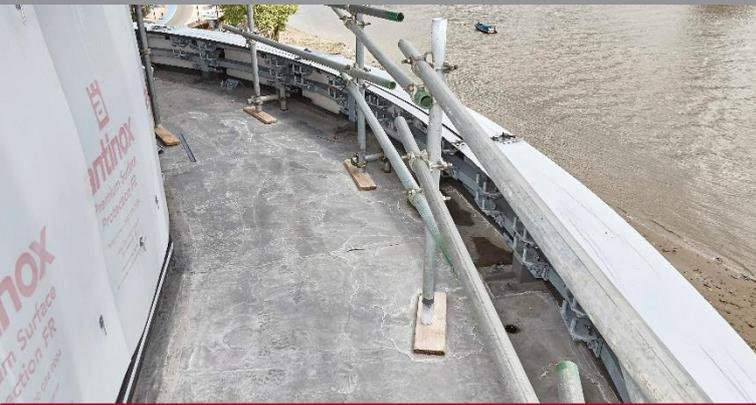
A sheet membrane solution would have been excessively complicated, whereas a liquid becomes homogenous. The AH 25 waterproofing would be hidden behind the cladding; so roofing contractors, Knight Asphalte had to be confident in its performance.
