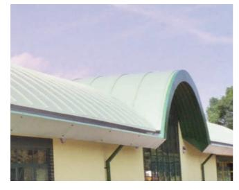
The **Rhenofol standing seam profile** is a hollow profile made of the same raw material as the roofing membrane, for installation on Rhenofol CV.
