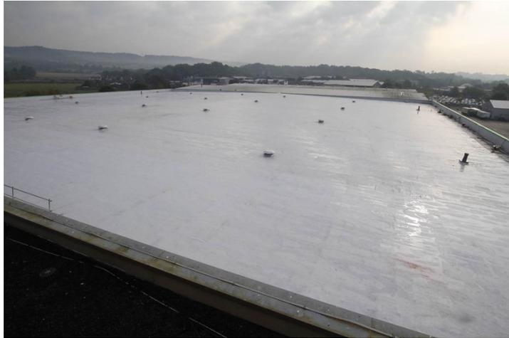
The roof to a Waitrose distribution centre has been completely refurbished in a single ply membrane system chosen for its sustainable credentials and no disruption to the retailer's 24/7 operations at Aylesford near Maidstone, Kent.
