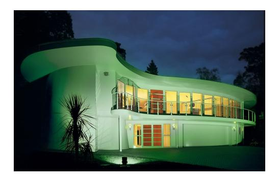
FDT's flagship "green" membrane, Rhepanol fk, was chosen for its unique, curvaceous roof. The bonded system was applied with Rhepanol Adhesive 90 and finished deftly with the contemporary copper coating to give it all the aesthetic qualities of traditional copper. Over time, the initial bright copper colour weathers to mellow bronze tones and eventually to a green patina.
