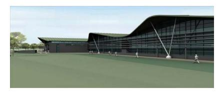
Armourplan PVC and Recticel Insulation by SIG Design & Technology were selected for a 12,000 m<sup>2</sup> roof to a bottling plant in a rural location on the outskirts of an historical Derbyshire spa town. The FMCG company chose to build the new facility away from the site of the natural spring, piping the water some two miles out of town to this green field bottling and distribution site.
