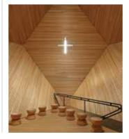
The 120mm thick plywood structural panels, while covered with Rhepanol and CorTen externally, are lined with larch internally.
