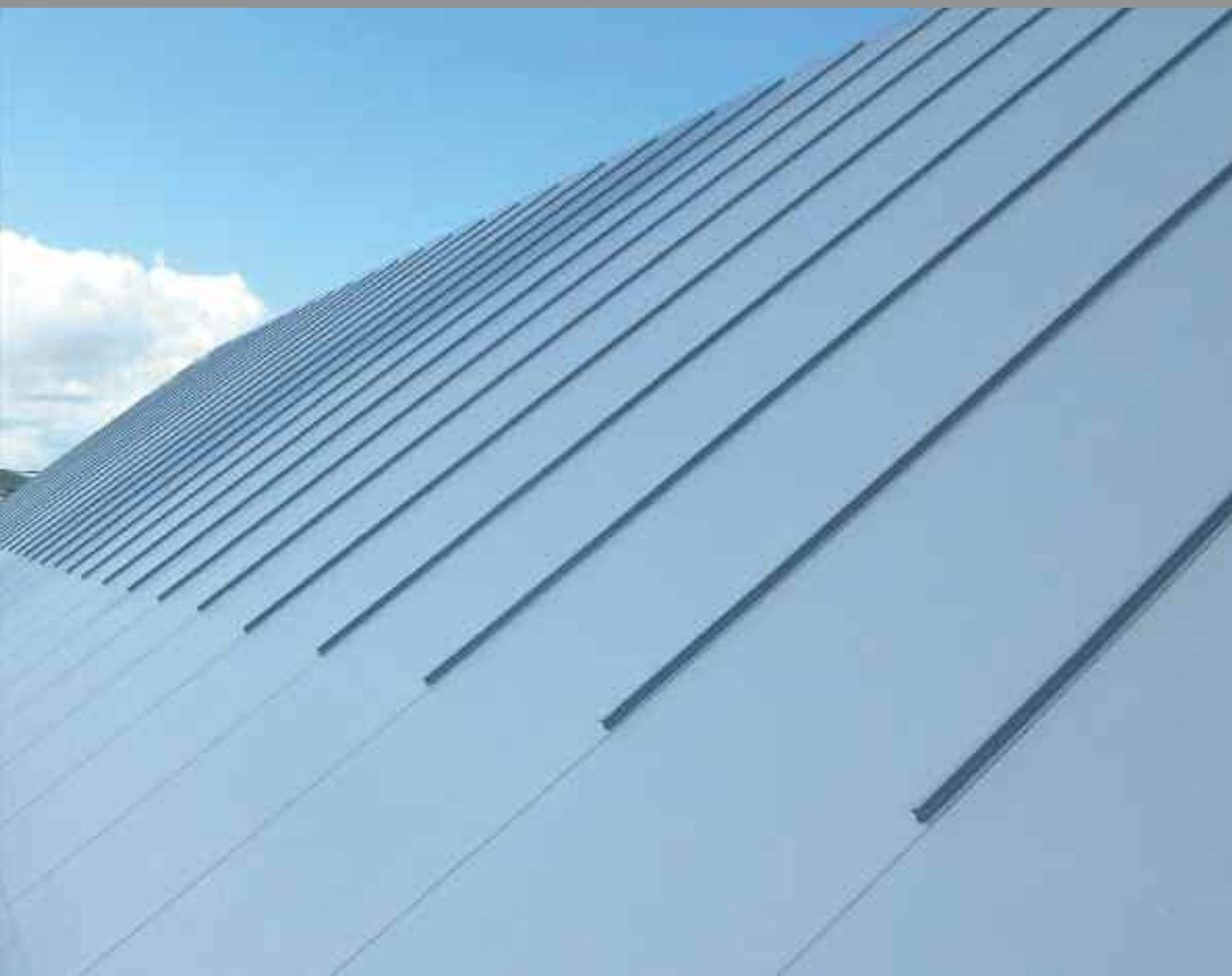
Armourplan is a PVC membrane that is produced at Clay Cross, Derbyshire, the only single-ply manufactured in the UK. It is suitable for use on a wide range of roofing applications including specialist installations such as simulated metal roofs.
