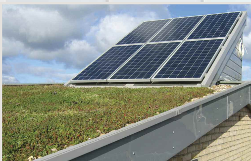
Blackdown's built-up green roofing system
