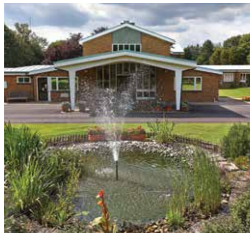
The use of Rhepanol fk roofing membrane finished with copper roof paint maintains the traditional appearance while dealing effectively with the threat of theft.
