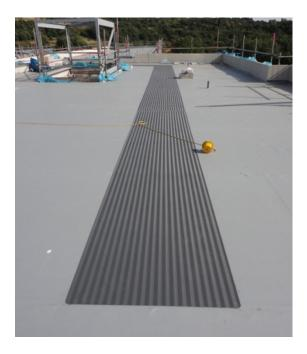
SIG became involved in the Discovery Academy project at a late stage to review the specification for the building's roofing system. The system was unusual in that it would omit the use of a screed, and instead mechanically fix the insulation and single ply membrane direct to the pre-cast concrete beams that had been laid at a 1:40 fall.
