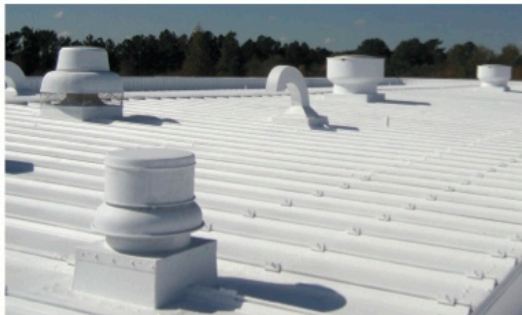
Top: Fletcher Rae Architects chose IKO Armourplan Premium PVC for its Buxton bottling facility in the Peak District. Above: Hot melt waterproofing on zero falls was installed at Riverbank House in the City of London. Left: A cold, liquid-applied waterproofing system was specified to refurbish this metal-decked plant room.
