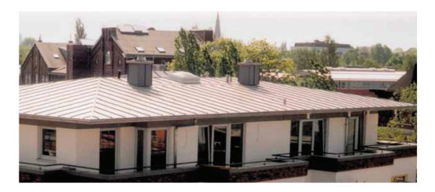
The **Rhenofol standing seam profile** is a hollow profile made of the same raw material as the roofing membrane, for installation on Rhenofol CV.
