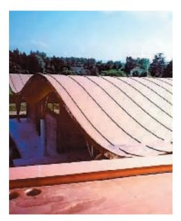
The Rhepanol fk standing seam profile is a solid polyisobutylene profile with a prefabricated self-sealing edge for installation on Rhepanol fk.
