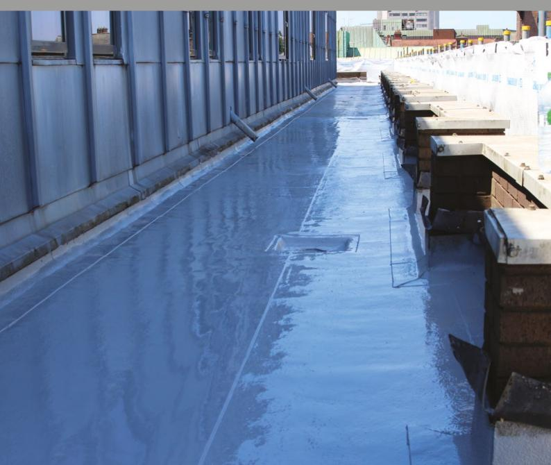
A revolutionary, fast curing, pure elastomeric, hydrophobic, polyurethane flat roofing system. SIGnature PU Liquid Coatings can be applied as a single coat (PU-20 Kit with accelerator component added) with only localised reinforcing as required, creating a bubble-free and durable liquid applied roofing system.
