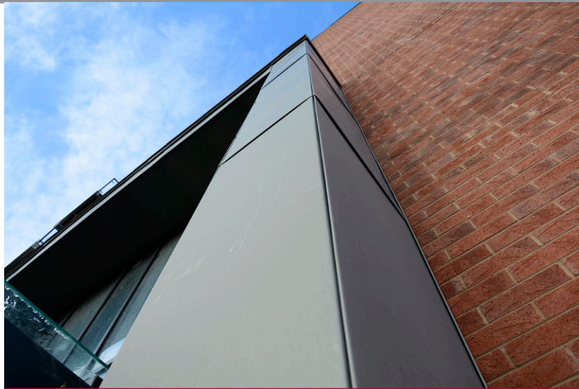
Crisp flatlock joints in the entrance canopy of the development
