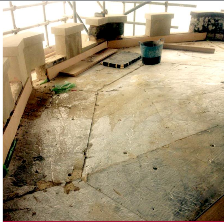
AH-25 was used as an alternative to lead - traditionally used on buildings of this age - due to its ability to be used on a shallower pitch.
