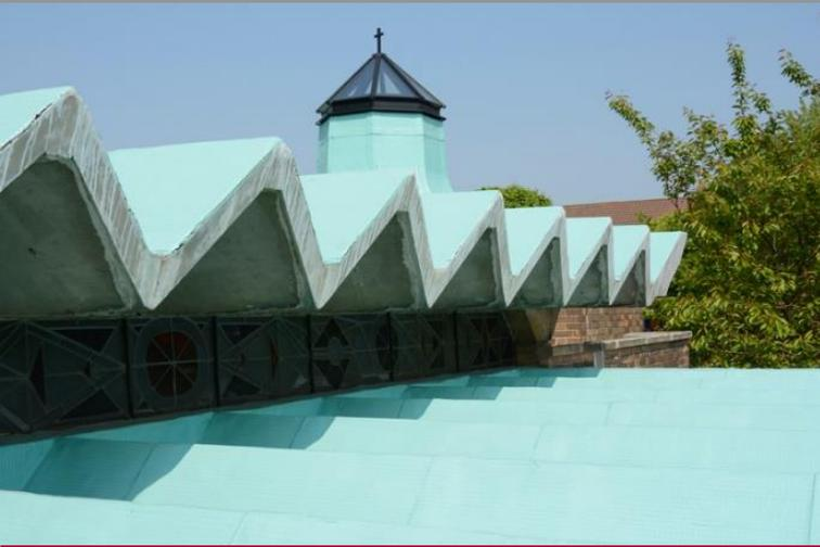
The existing bitumen covering had bonded with the concrete making it impossible to remove without damaging. Repoma can waterproof almost any roof surface without removal.
