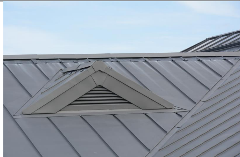
The new roofs were installed on the first ward block in a 10-month period with no disruption to the patients
