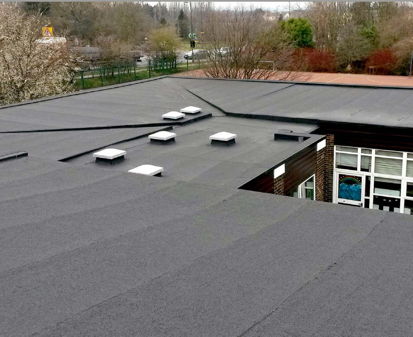
An EXT.F.AA fire rated roofing system intended for both new work and overlay projects. Offering different warranty packages dependent on the underlay option selected. This will ensure that you can tailor the system to your client's requirements, and come in on budget.
