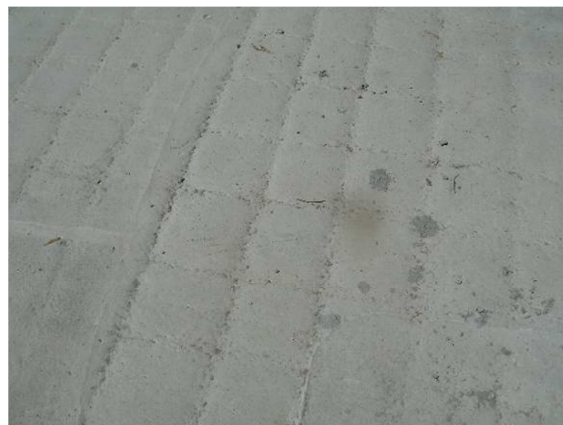
Figure 2 – example of 'reinforcement ripple'
