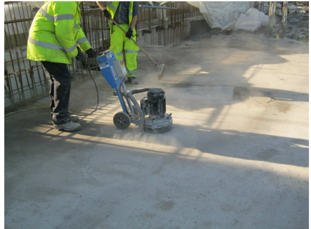
Figure 5 – removal of surface laitance
