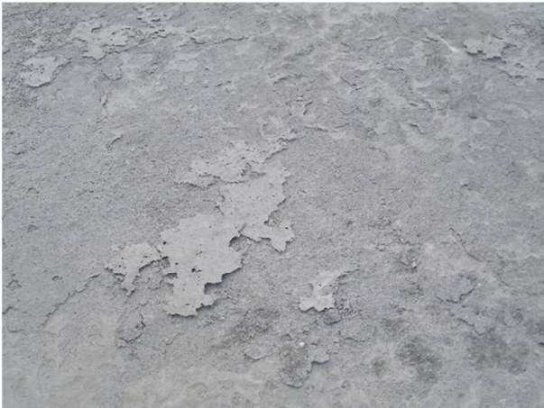
Figure 3 – example of surface laitance
