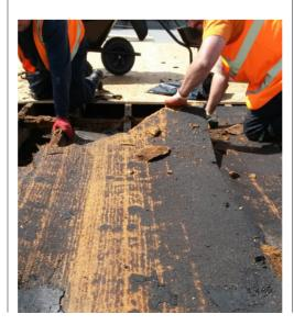
**Bottom** A school roof refurbishment in Glasgow: over 90% of the roof was damaged. **Below** Condensation between layers causing delamination.
