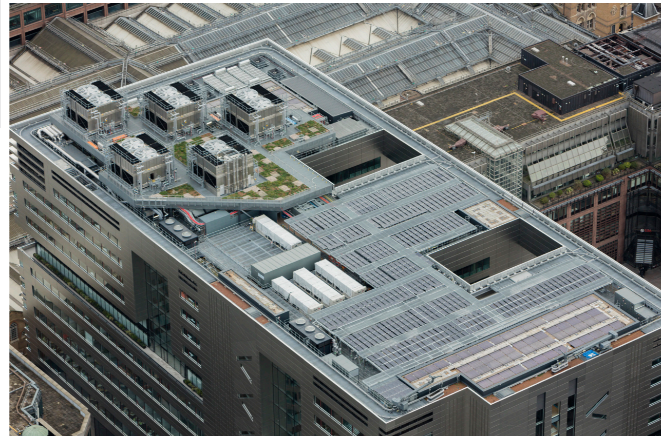
Above: Hot melt was right for the complex roof at UBS' Broadgate HQ.
