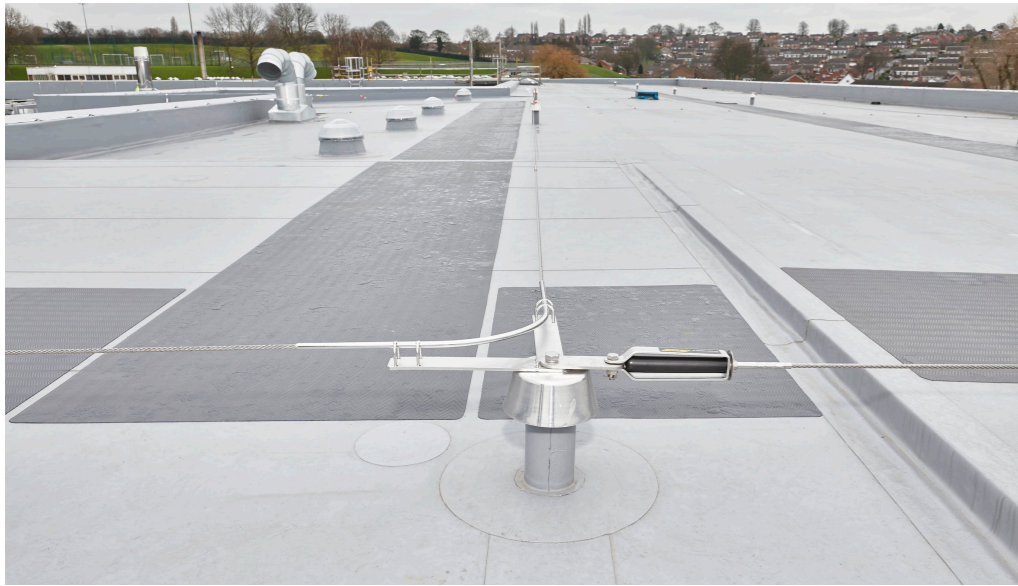
Above: Single ply roof at Arnold Hill Academy, Nottingham.
