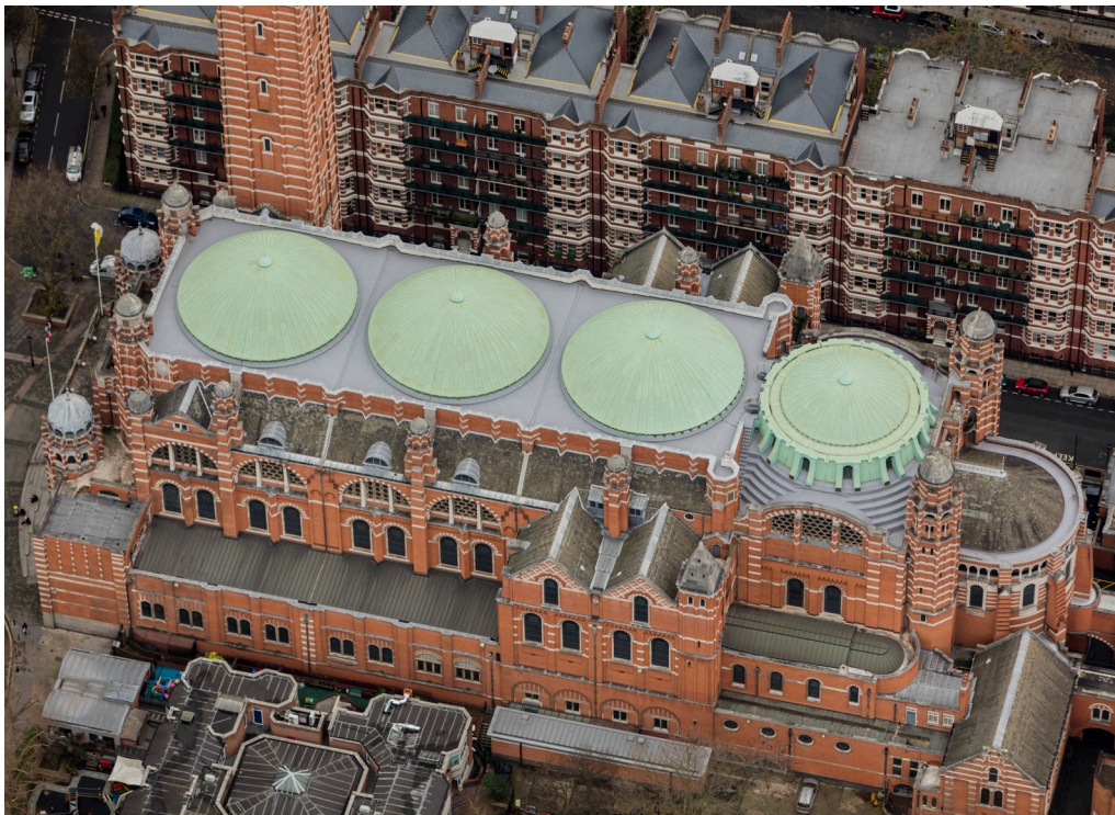
Left and below Abutments to the copper domes and brick parapets were the biggest challenge.
