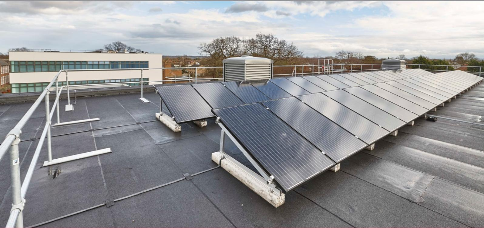
deck, the bitumen primer required for the felt vapour control layer would stain the decking webs and with no ceiling, this would be unsightly. SIG negotiated a hybrid system with our partnering manufacturer comprising a robust, cost effective, reinforced bituminous membranes with a polyethylene VCL to solve acoustic and aesthetic issues.
