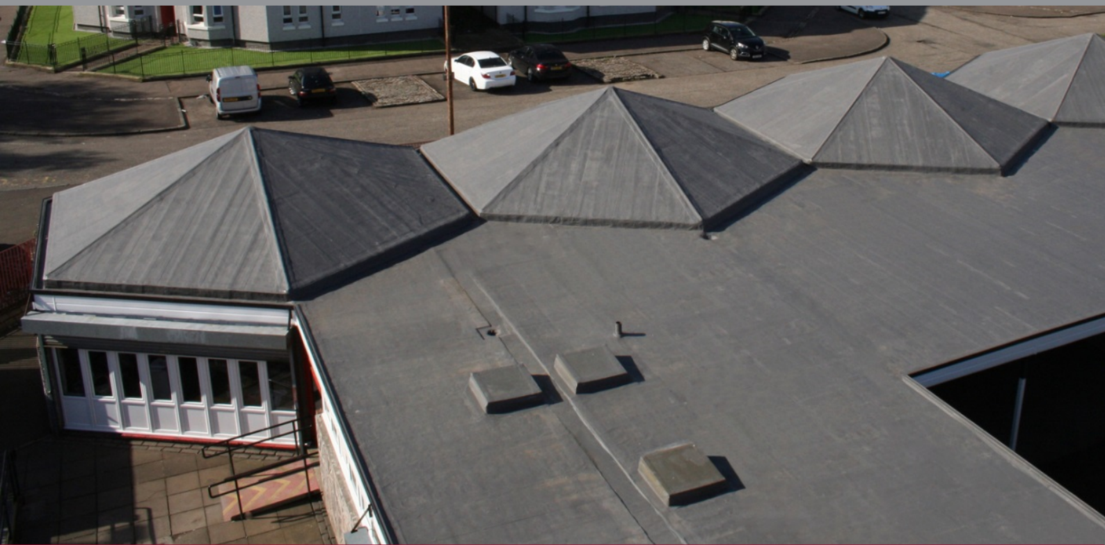
Sacred Heart Primary School, Glasgow 450m 2 of roof refurbished in Hydrostop AH+
