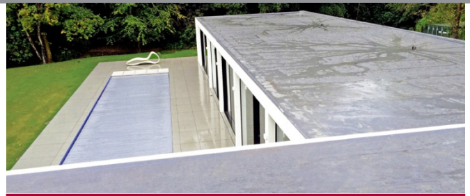
IKO Armourplan P PVC Single Ply Membrane flat roof application illustrating the clean uncluttered finish.
