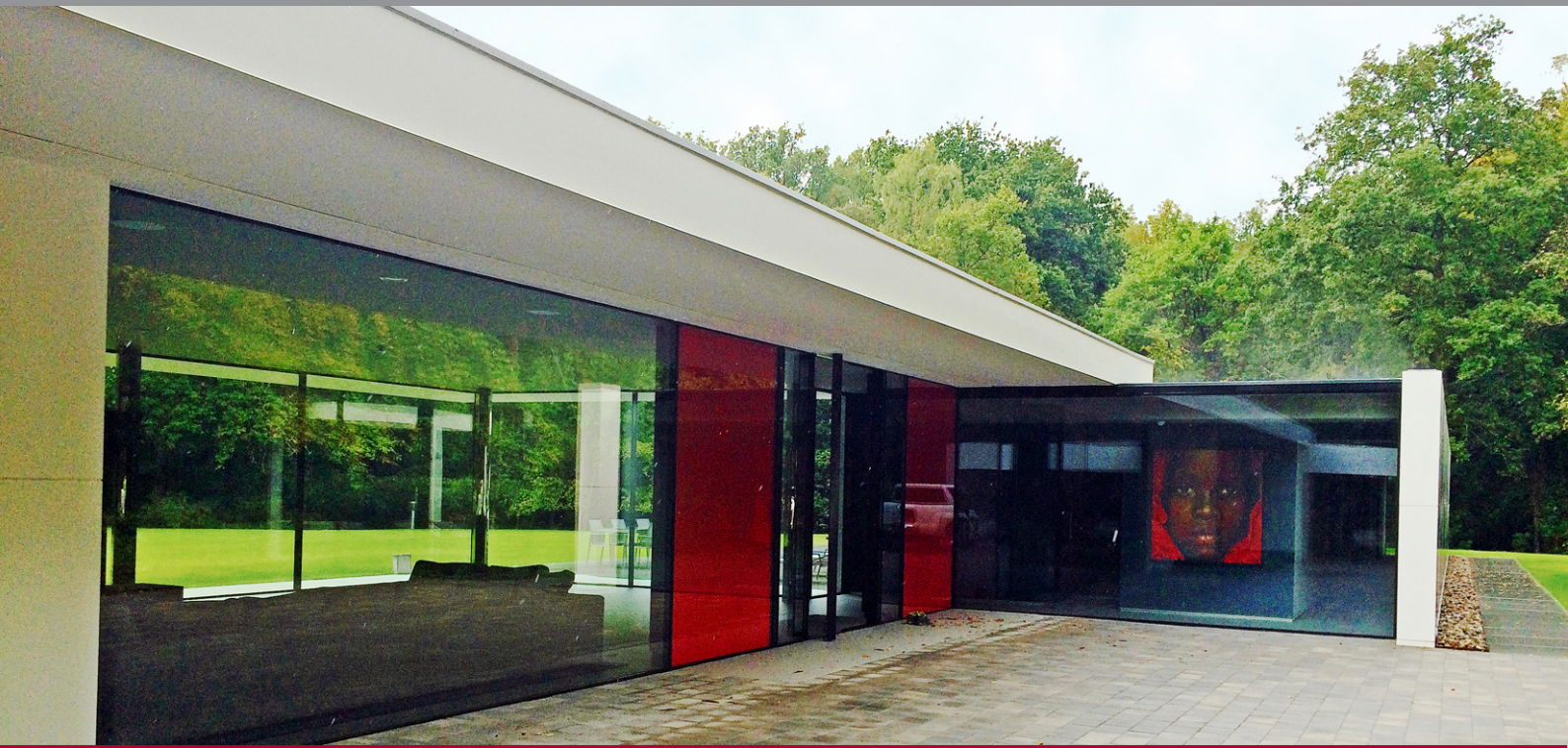
Front elevation of the property showing the minimalist requirement for the flat roof application
