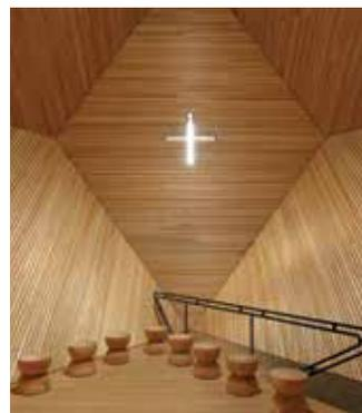
The 120mm thick plywood structural panels, while covered with Rhepanol and CorTen externally, are lined with larch internally.
