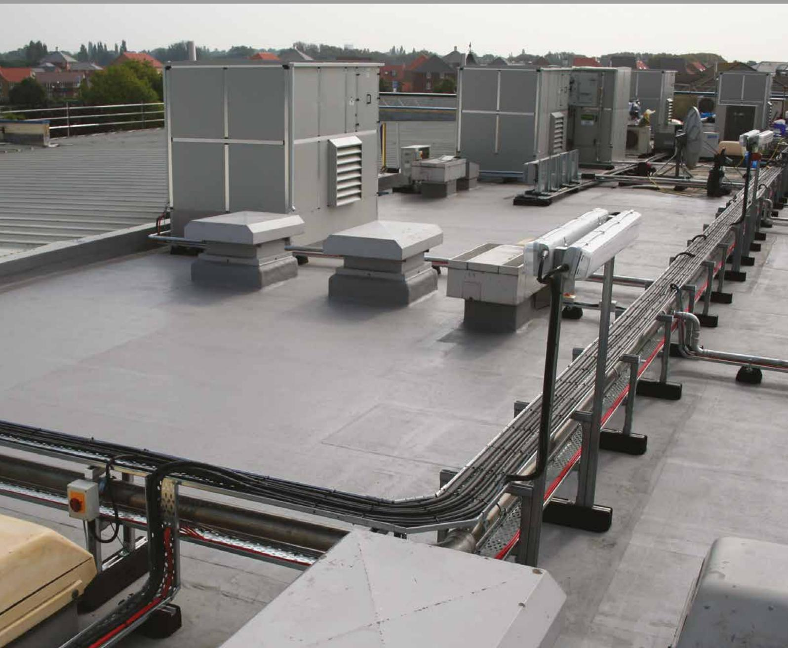
**AH-25** is a one-component liquid waterproofing system which offers significant advantages over conventional PU and PMMA systems. It is fully reinforced with a polyester fabric and cures quickly – it can be applied under practically any conditions, even on cold days and on most surfaces.
