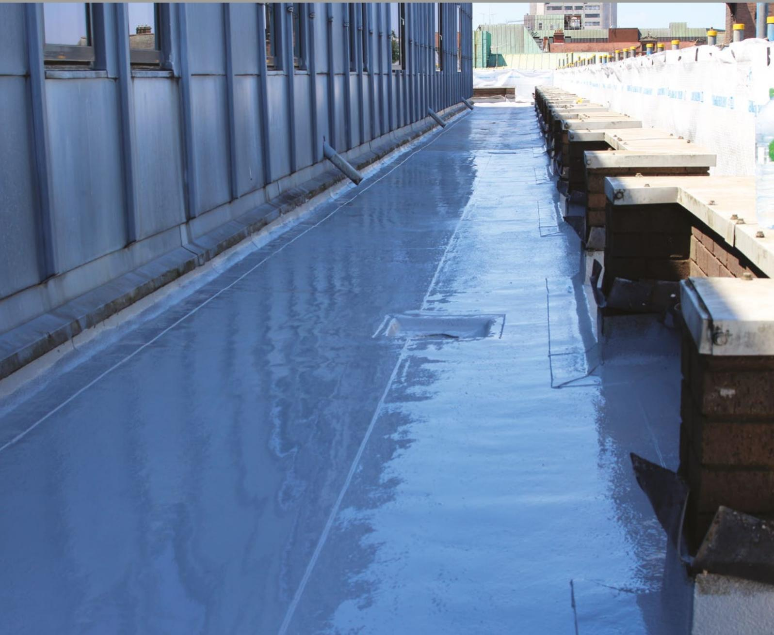
A revolutionary, fast curing, pure elastomeric, hydrophobic, polyurethane flat roofing system. SIGnature PU Liquid Coatings can be applied as a single coat (PU-20 Kit with accelerator component added) with only localised reinforcing as required, creating a bubble-free and durable liquid applied roofing system.
